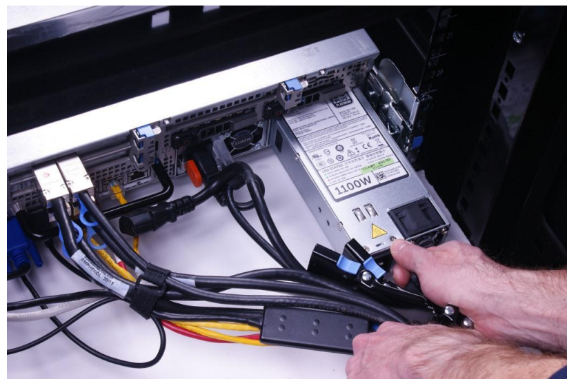
Figure 8. Replacing the outer power supply
